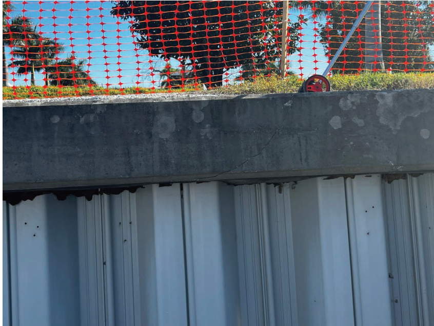
Photo #4 – View of Settling and Movement of Seawall.
