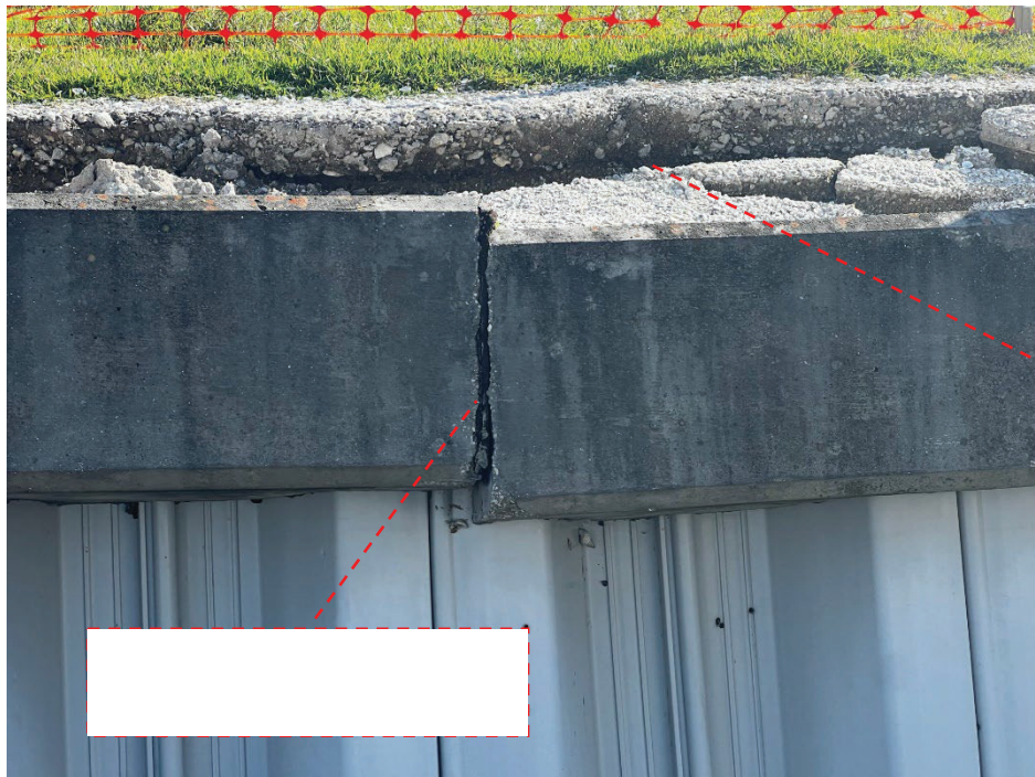
Photo #4 – View of Settling and Movement of Seawall.
